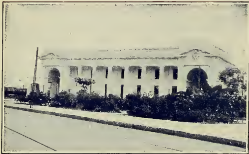
The Panama Railroad Station, Panama City
